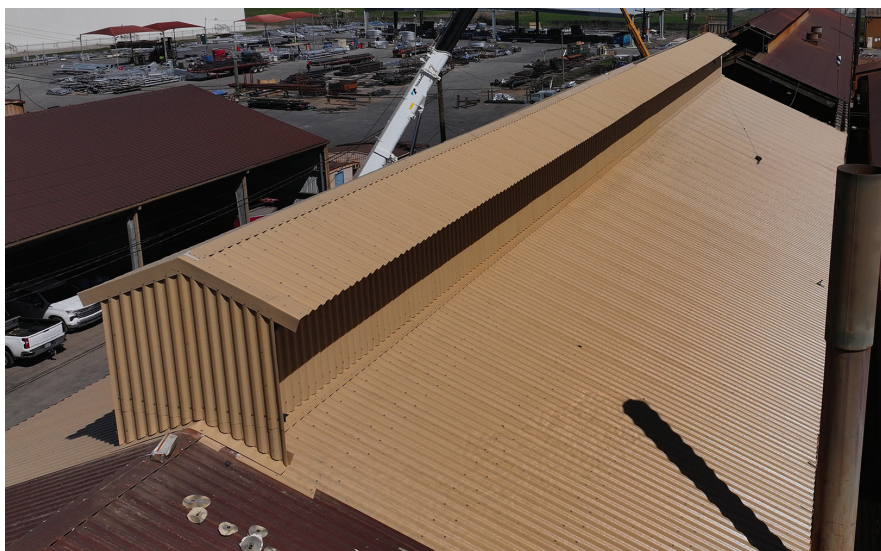
Roof with Enduro Composites panels installed.
