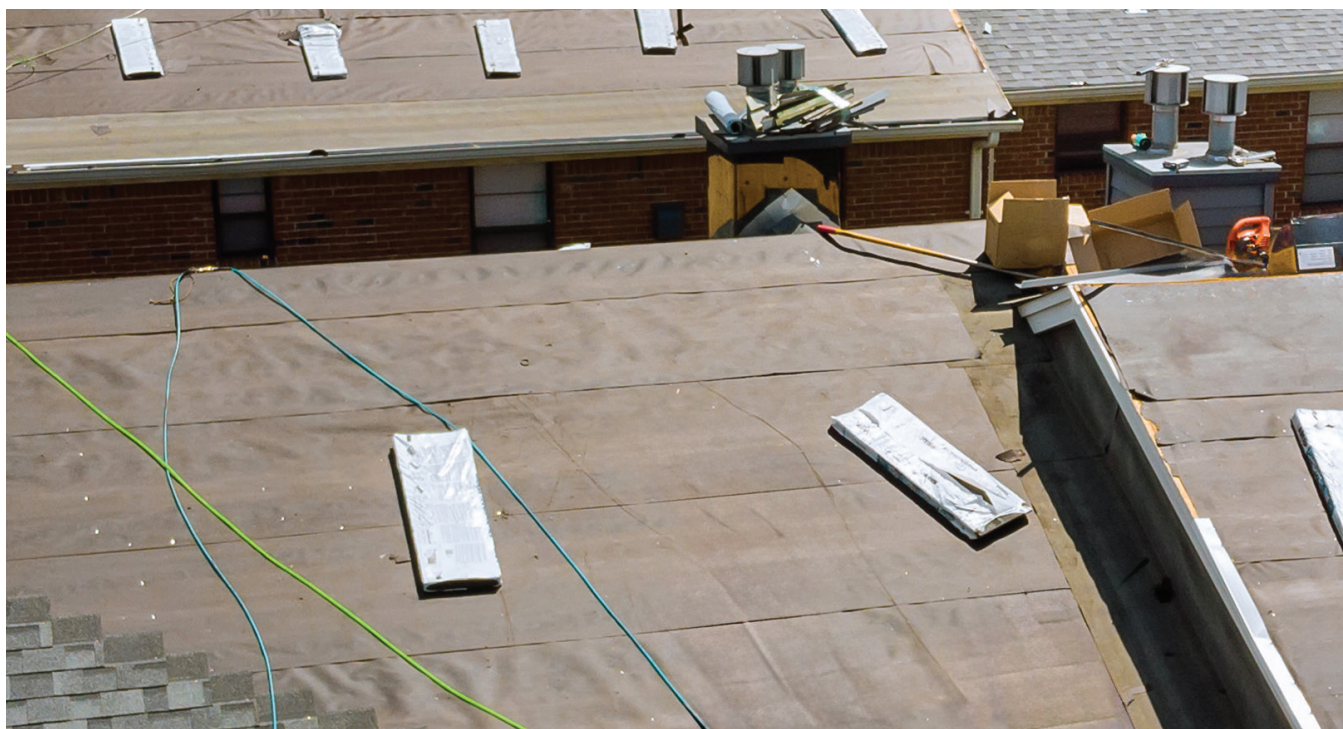
Keep shingles in packaging until they are ready to be applied.
