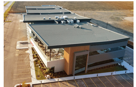
GPD Flatroofing Ltd. – Penn-co Office Steinbach (Steinbach, Manitoba)
