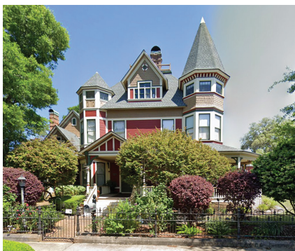
Stonebridge Roofing, Energy & Exteriors – The Bailey House (Fernandina Beach, Florida)
