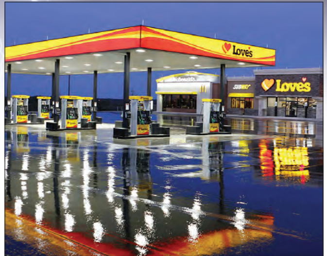
A high lightning risk assessment resulted in the installation of a lightning protection system on the store and fuel canopies. Images courtesy of East Coast Lightning Equipment Inc.
