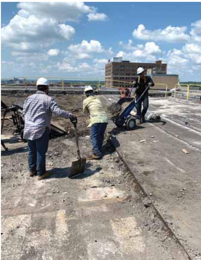
Western Specialty Contractors workers installing new Hydropack roof garden system. Photo courtesy of Western Specialty Contractors.
