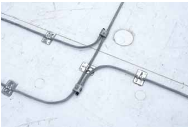
Lightning protection standards contain specific requirements for conductor coursings, fastener placement and interconnection methods for joining conductors and building systems. Photos courtesy of East Coast Lightning Equipment, Inc.
