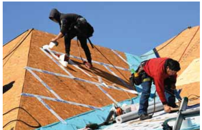
When putting a roof on a new or existing home, Fortified requires sealed roof deck seams, among other requirements. PHOTOS COURTESY OF IBHS.
