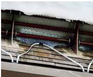
A heated cable system assists with roof and gutter de-icing. PHOTO COURTESY OF FLOTRACE
