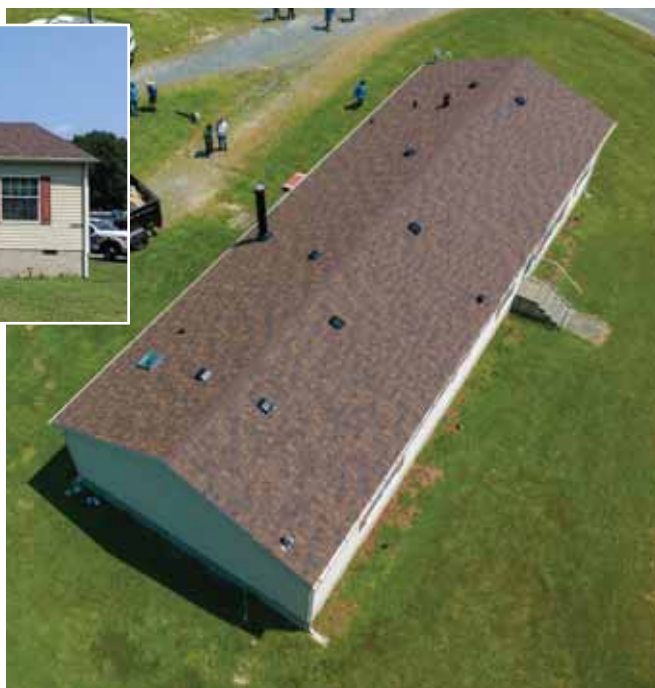
PHOTOS COURTESY OF ROOFPRO, SEVERN, MARYLAND.
