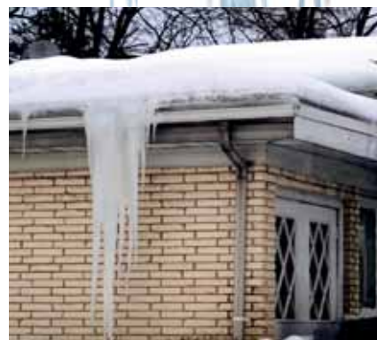
Large icicles have the potential to cause extensive damage and serious injury.
