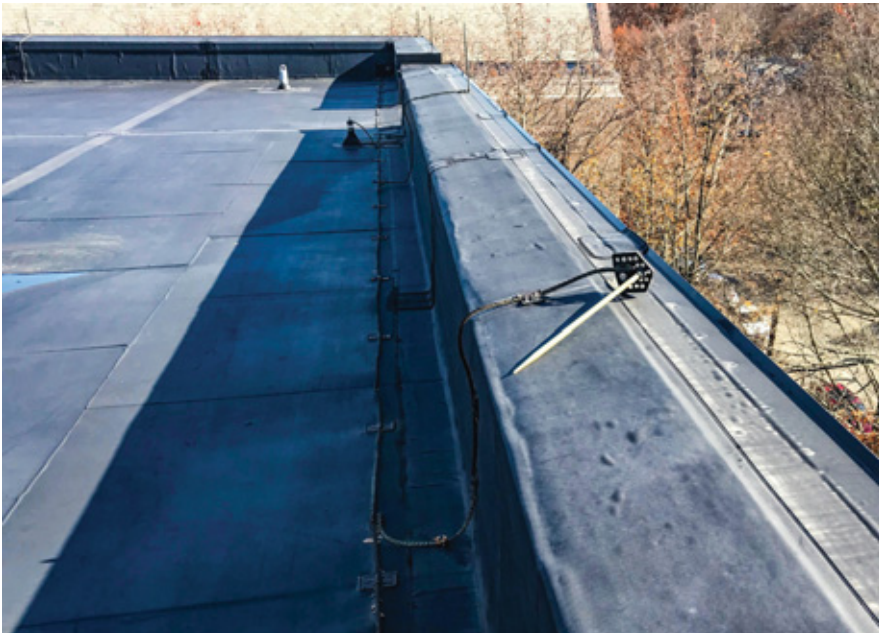
Neither the updated language, nor the referenced standards, address how LPS should be specially secured to existing roofing components, which led SPRI, Inc., the trade association representing the manufacturers of single-ply roofing systems and the related component materials, to take action to clarify how LPS components should be secured to edge metal and other roofing components.
