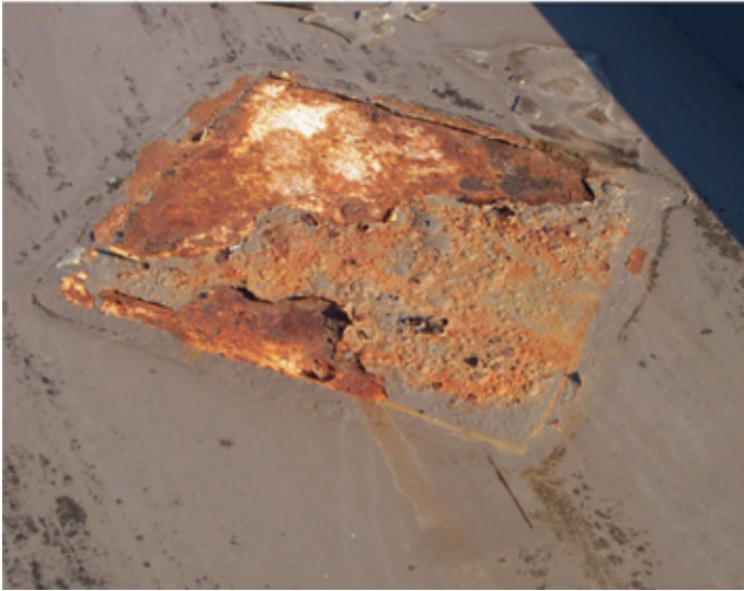
The adhesive bond is to paint. If the adhesive does not fail, the paint may fail, leading to corrosion.
