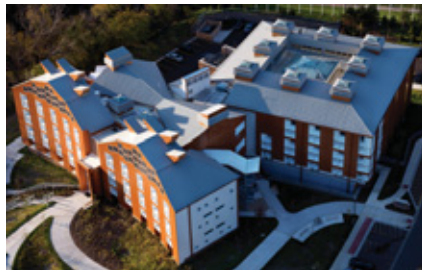
Medallion Lok standing seam panels from McElroy Metal grace the roof of Judson University, Elgin, Illinois.
