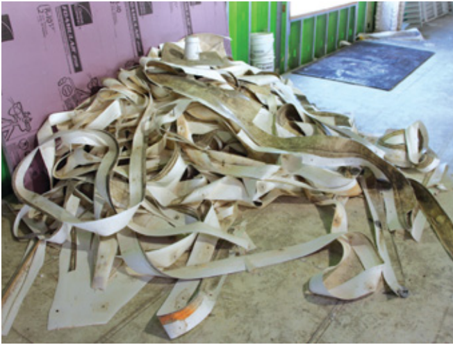
More than a million pounds of PVC are being converted into new membrane and other non-roofing products annually. PHOTOS COURTESY OF CFFA.
