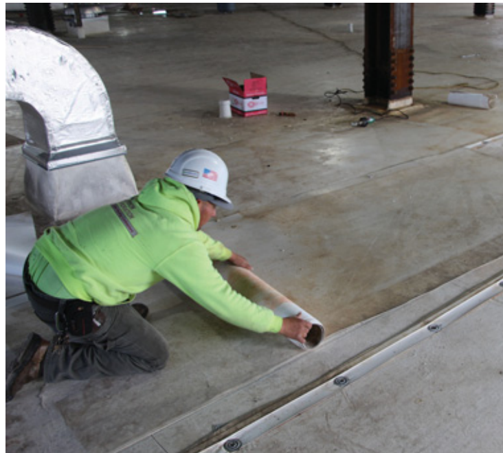
During removal, PVC should be rolled for easier handling.
