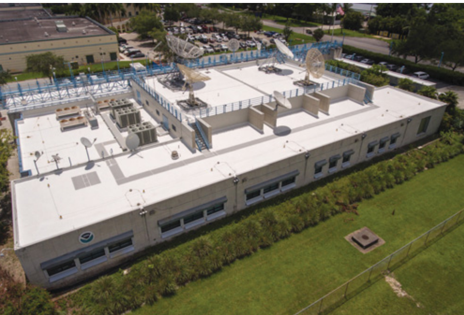
The National Hurricane Center of the National Oceanic and Atmospheric Administration (NOAA), located in Miami, has a PVC roof. The roof weathered Category 4 Irma without failing.
