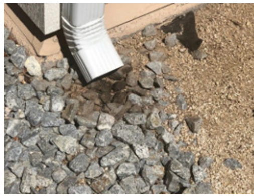
Staining on landscaping (discoloration of aggregate). COURTESY OF POLYGLASS/S. WADDING
