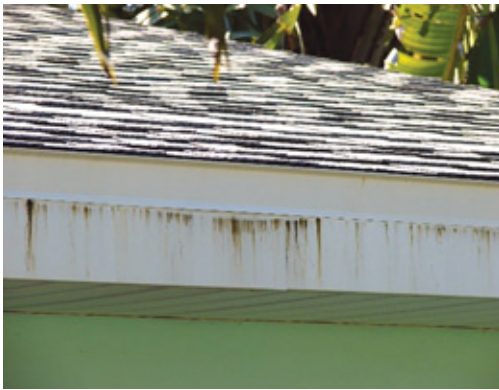
Staining on trim. COURTESY OF OWENS CORNING
