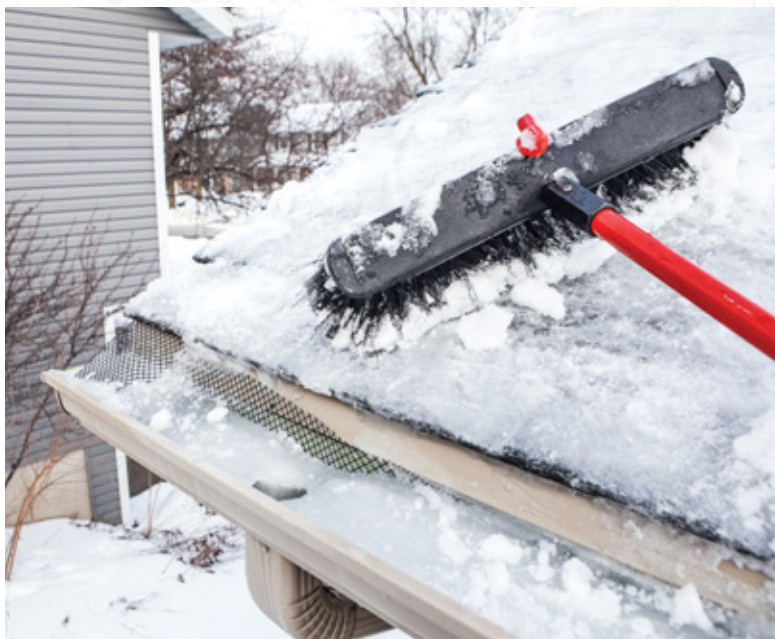
Ice buildup at the eaves can cause severe damage.
