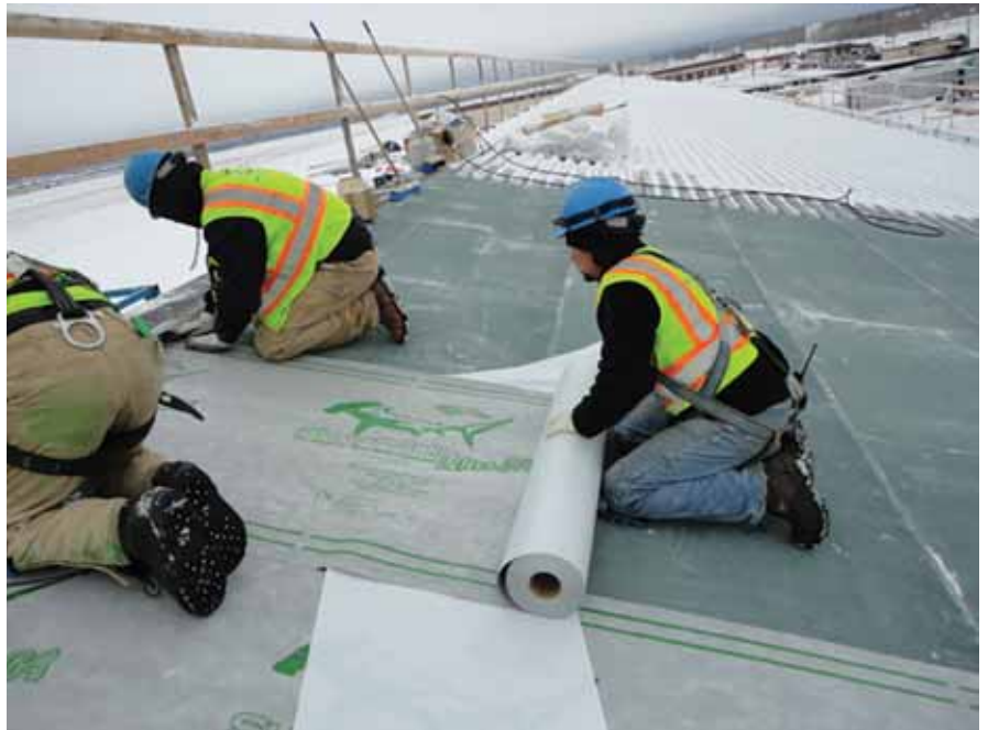
Sharkskin Ultra SA® installed over DensDeck. Fort Wainwright, Fairbanks, Alaska. This underlayment sticks in the cold – down to 10°F – without primer.
