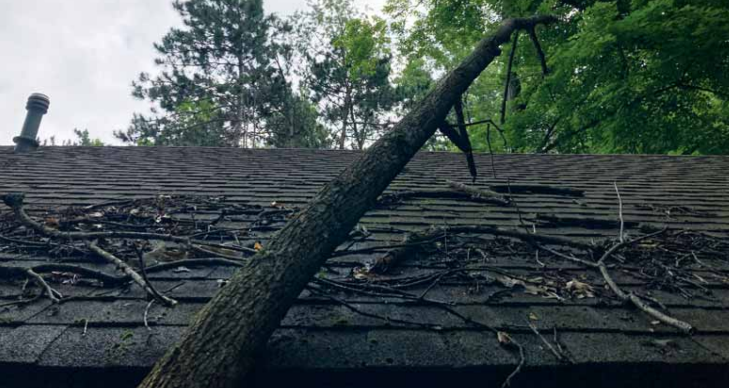
The hazards of wood and roofs extend beyond damage from falling trees and branches. Debris such as leaves and branches provide organisms with moisture, an added place to grow, and possibly even nutrients.
