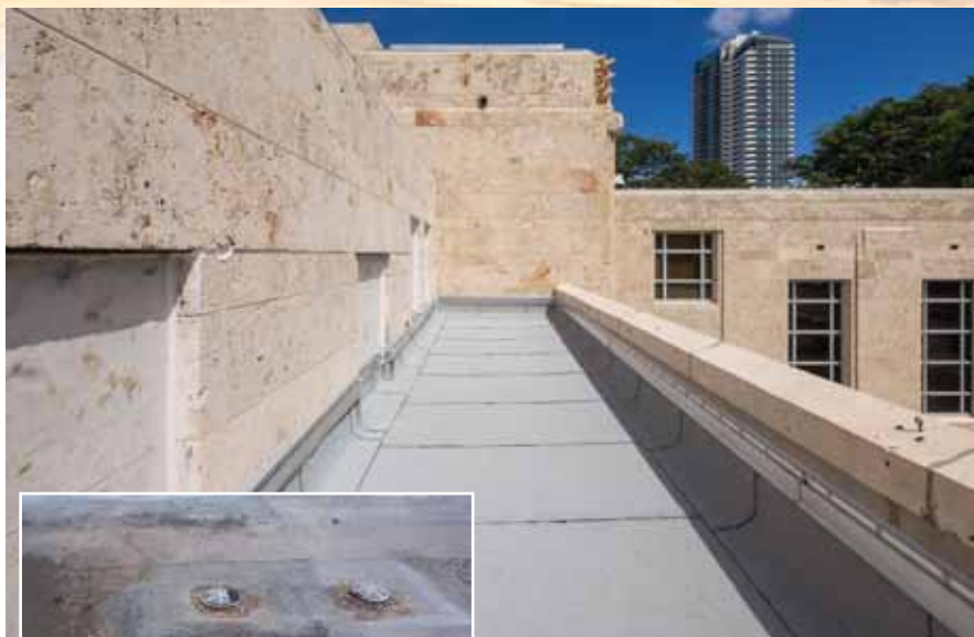
Above: The Bass Art Museum holds up to South Florida's intense heat with a premium capsheet designed for superior mineral retention.
