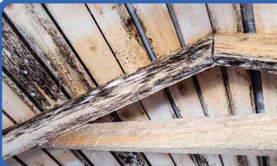
Inspect attics for mold and other problems. Be sure to report all findings to the homeowner.
