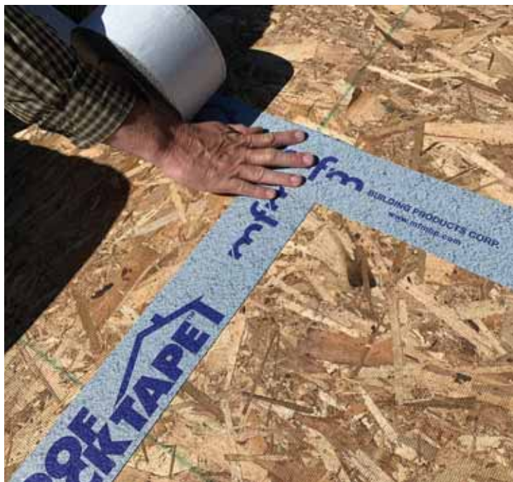
As you work across horizontal seams, be sure the membrane completely covers the ends of the membrane installed on the vertical seam sections.
