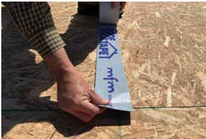
Start by rolling the vertical seams, making sure to fully intersect the horizontal seams.
