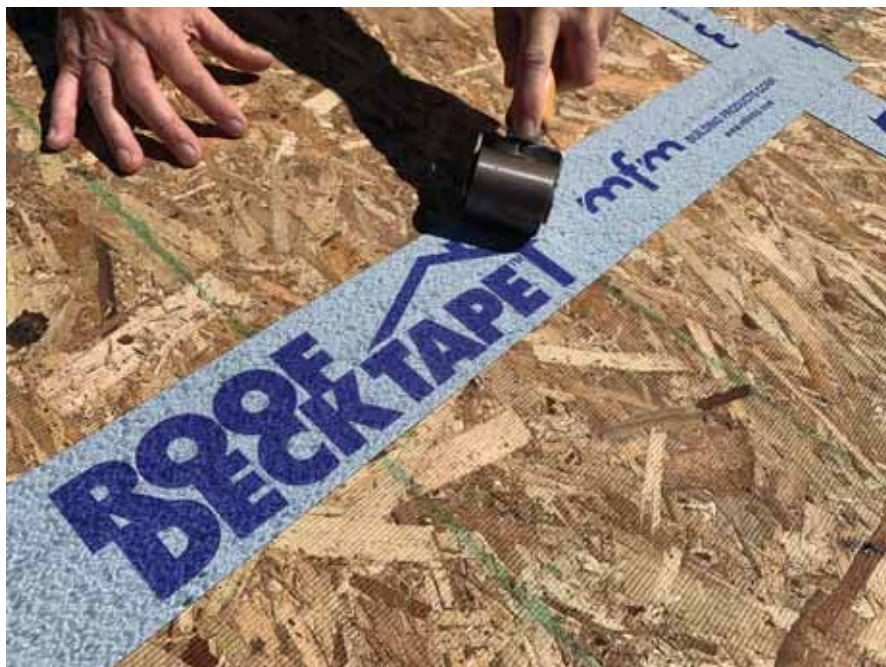
Roll the entire membrane thoroughly with a hand roller to ensure maximum contact of the adhesive system to the substrate. PHOTOS COURTESY OF MFM BUILDING PRODUCTS
