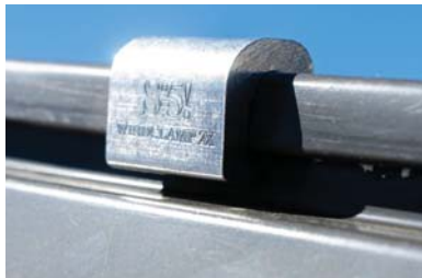
Selected clips need to meet or exceed the wind uplift requirements for every unique building. Photo courtesy of S-51
