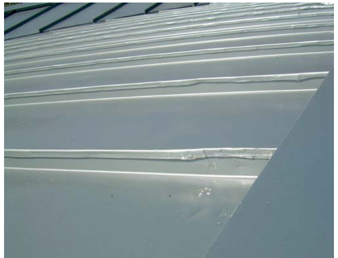
Top, Above, and Right: “How not to repair a roof”—some previous repairs can give you an idea of what you’re in for when you get up on the roof. Photos courtesy of Petersen.
