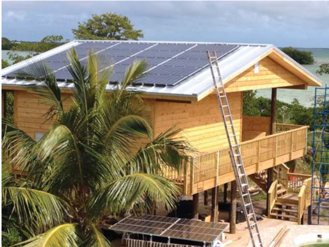
Above: This building survived Hurricane Irma, with a roof design capable of withstanding 180 mph winds. Photo courtesy of S-5I
